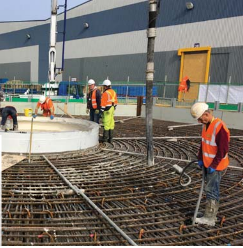
CEMEX was the 2019 winner for this wind turbine base.
