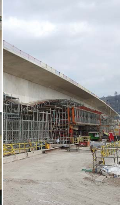
Medway River Bridge.
